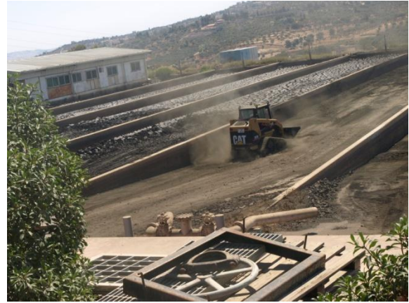
Figure 1 – left: the sludge bed is filling up, right: a front-end loader is taking the dry sludge for fertilizer
